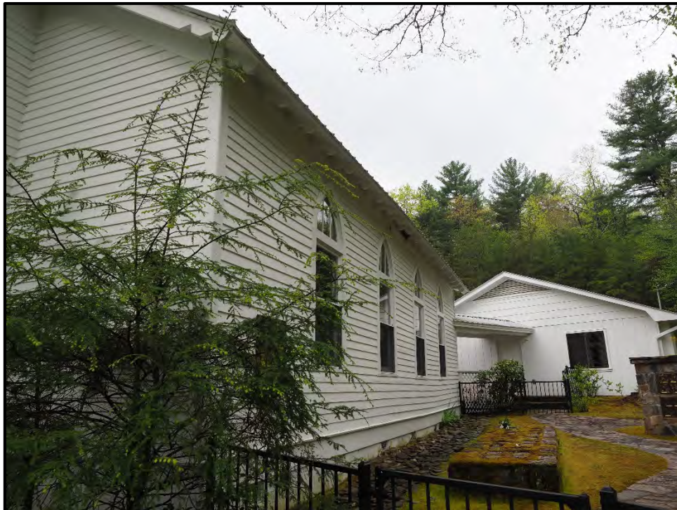
Figure 38: Lake Toxaway Methodist Church, side elevation and rear addition.
