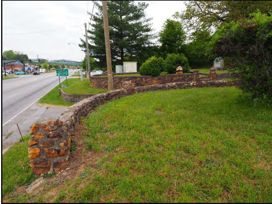
Figure 27: Stone walls constructed of river rock flanking the entrance drive.
