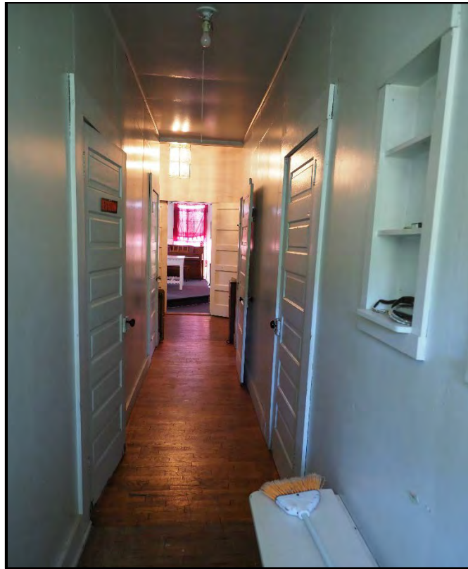
Figure 24: Detail of addition hallway looking towards the sanctuary.
