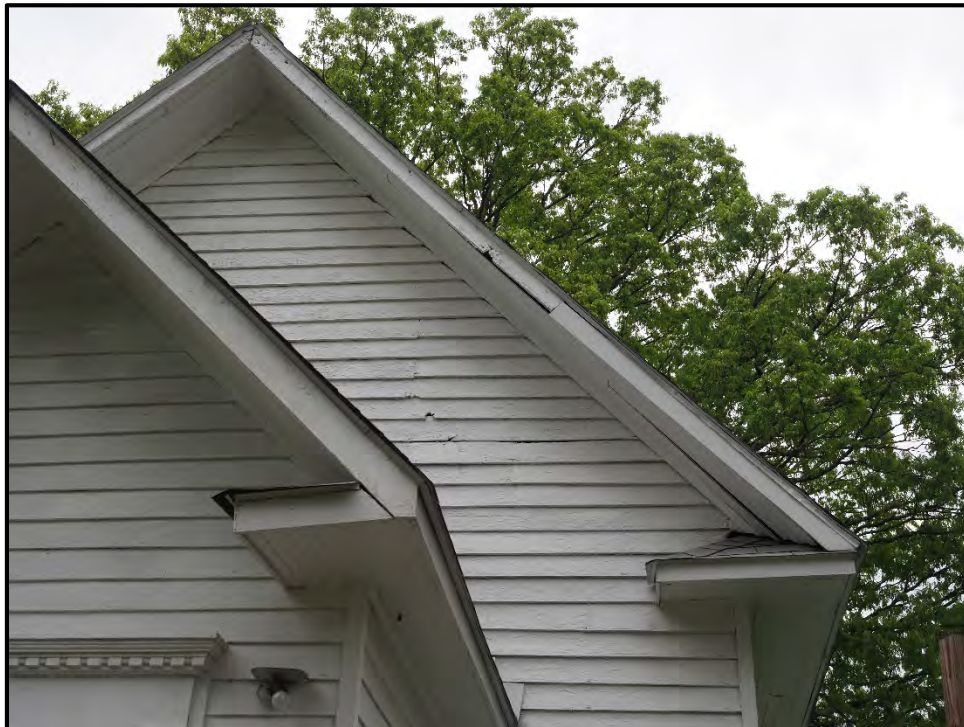
Figure 12: Detail of front façade with moldings and end-returns.
