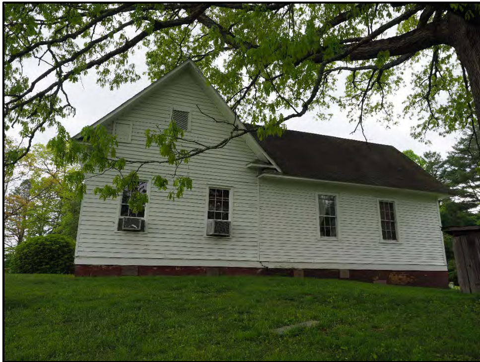
Figure 10: The church's northern elevation with double gable end returns.
