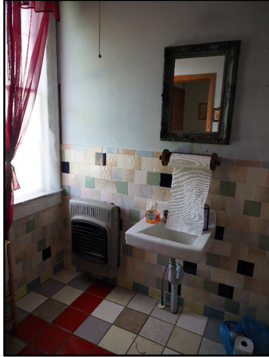
Figure 23: Detail of bathroom sink and mirror located in the church addition.
