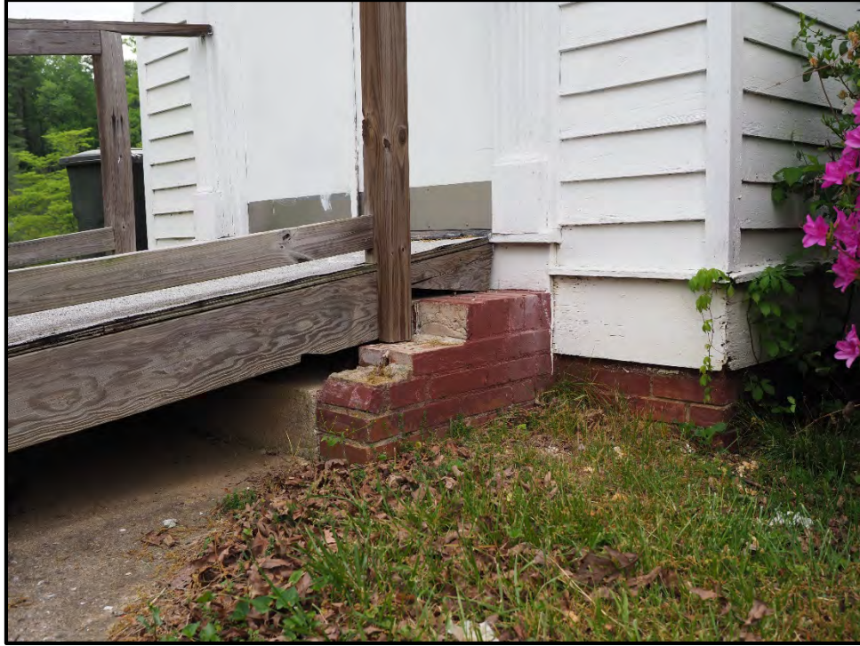
Figure 12: Detail of entrance stairs and modern wood accessibility ramp.
