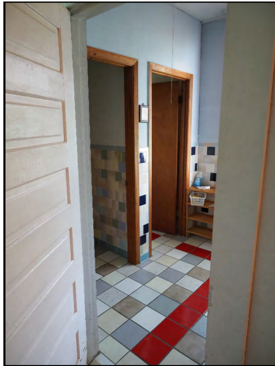
Figure 22: Detail of entrance to bathroom in the church addition.
