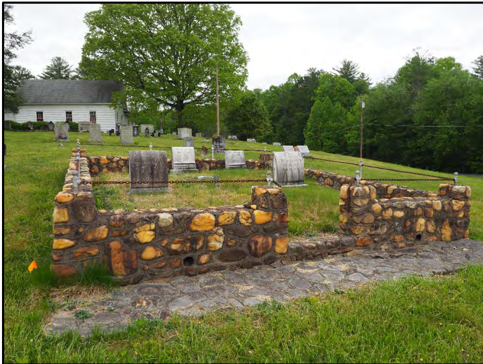
Figure 28: Example of stone wall constructed of river rock surrounding a family burial plot.
