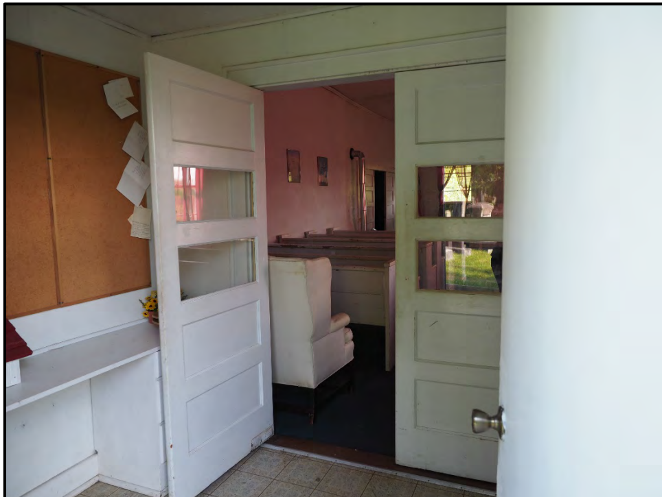
Figure 16: Detail of vestibule with original five-panel doors.
