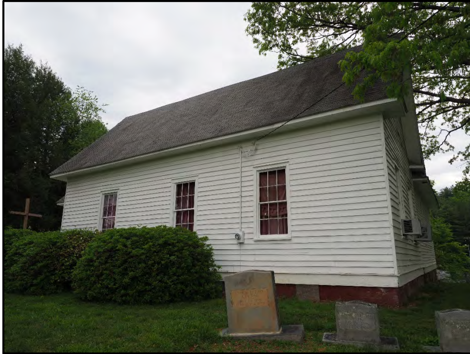
Figure 11: Side elevation of the church, looking west.
